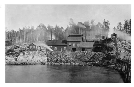
Everyone woke up to a surprise one morning in December, 1956, when they discovered that Texada Mines' 500-foot wharf and loading dock were missing! The pilings rested on slippery tailings mixed with clay and the tidal pressure of a 60mph gale was enough to push it under in the night.
